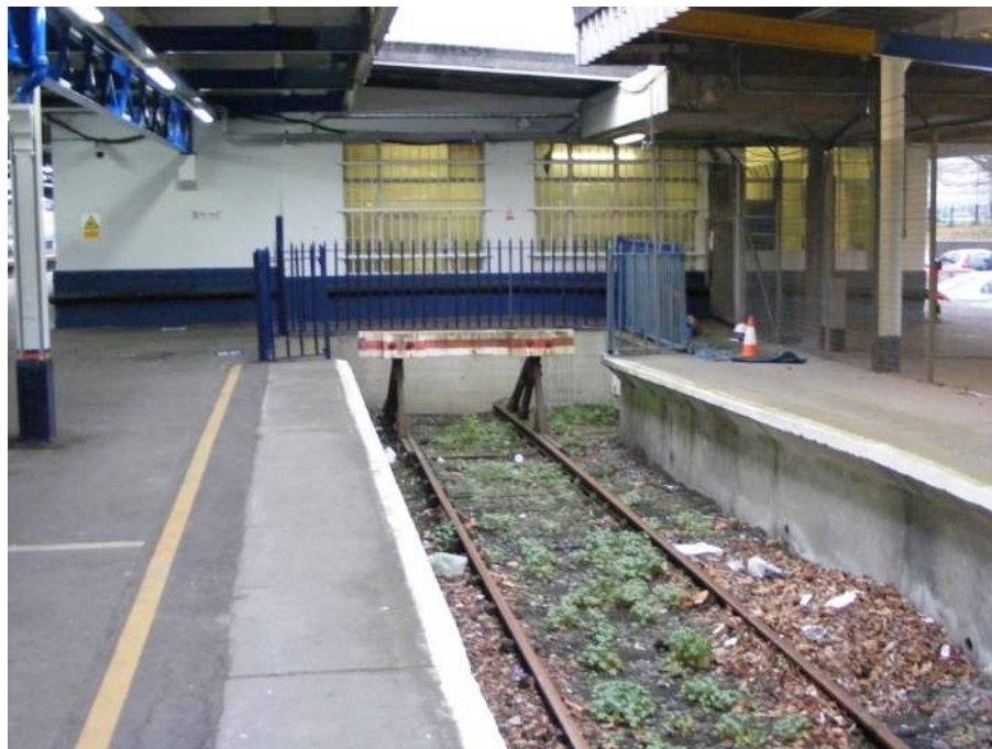
Figure 5 - Southampton Station existing buffer stop – to be shifted and re-used
