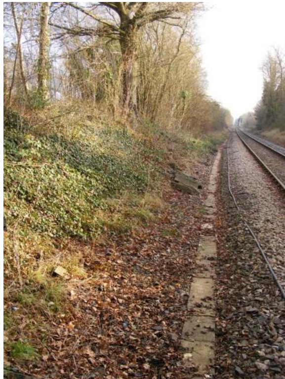
Figure 8 – Hounsdow proposed Station location looking south-east towards Jacob's Gutter Lane (northern side, required for both Option 1 and 2)
